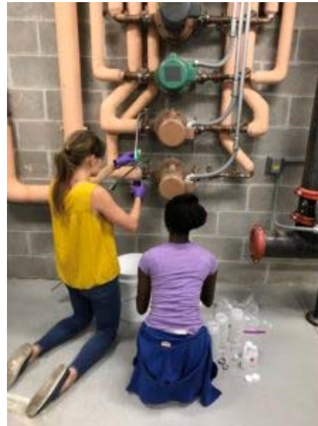
“New” water matrices: Premise Plumbing
